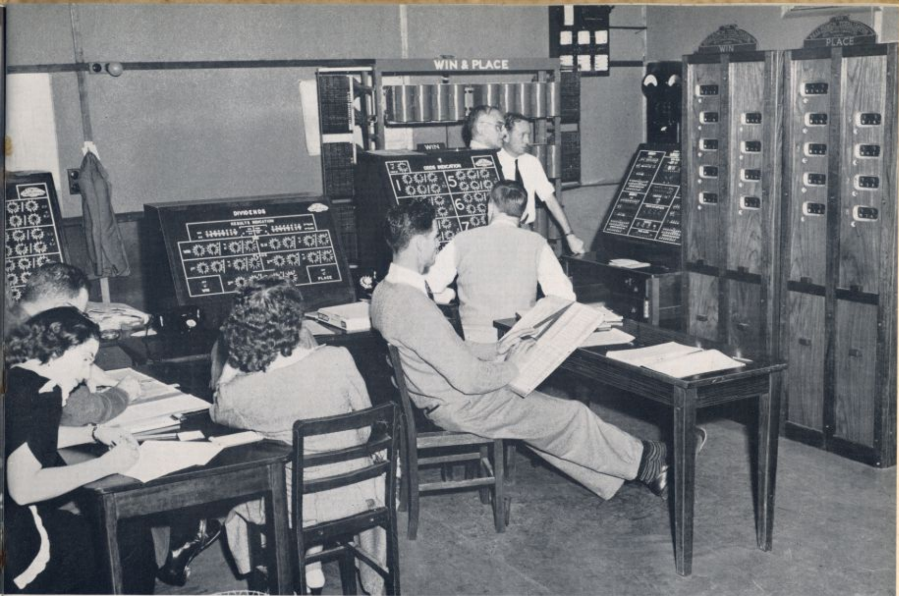
The Control Room
