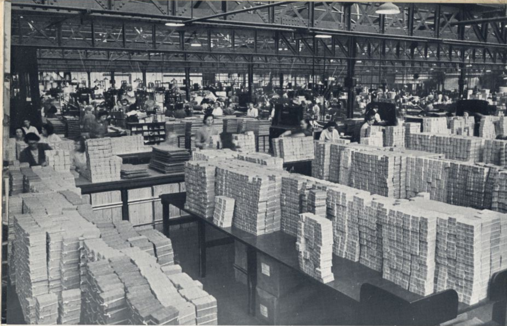
A DAY'S OUTPUT READY FOR DESPATCH
